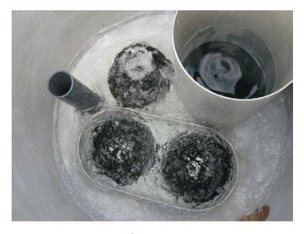
Figure 8 Top view photo of the Jellyfish<sup>®</sup> Filter JF4-2-1 during operation. Filtered water exits the cartridge lid orifice as a pulsating fountain.
