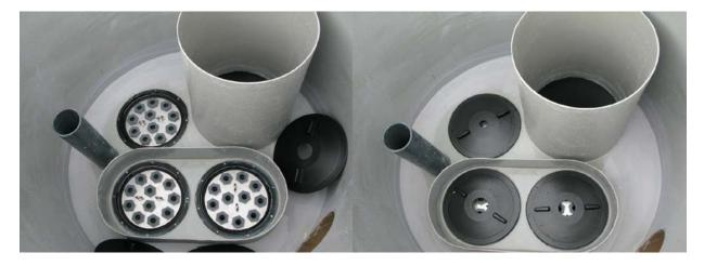
Figure 7 Top view photos of the Jellyfish<sup>®</sup> Filter JF4-2-1 deck with two hi-flo cartridges and one draindown cartridge installed with cartridge lids off (upper left image) and cartridge lids on (upper right image). The backwash pool weir encloses the hi-flo cartridge. Also shown are the maintenance access pipe (large), pressure relief pipe (small), and the outlet opening (lower right in each image).
