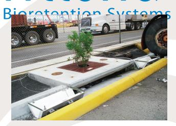
Filterra<sup>™</sup> monitoring unit at a port.
