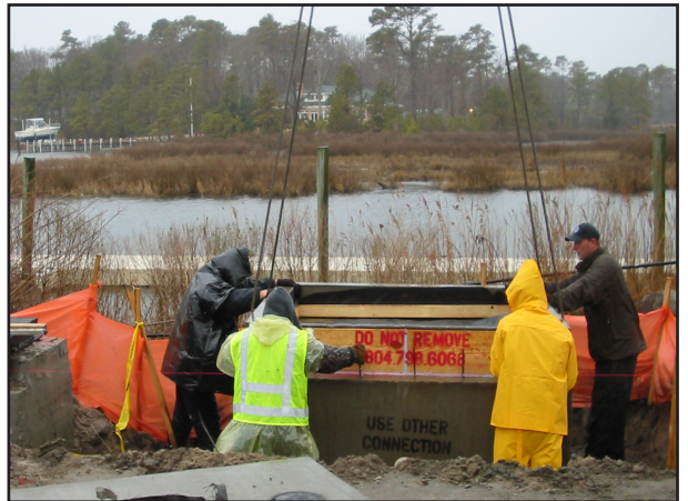
4. Manufacturer-installed protective throat board and internal silt fabric must be left in place to protect the unit from construction sediment. The top slab is set with butyl tape seal (also supplied).
