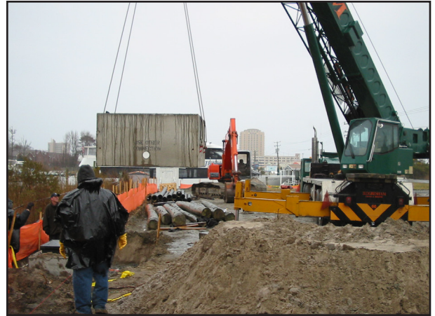
2. A crane is used with a spreader bar or long slings to unload and set the units. Box is lifted separately from top slab.
