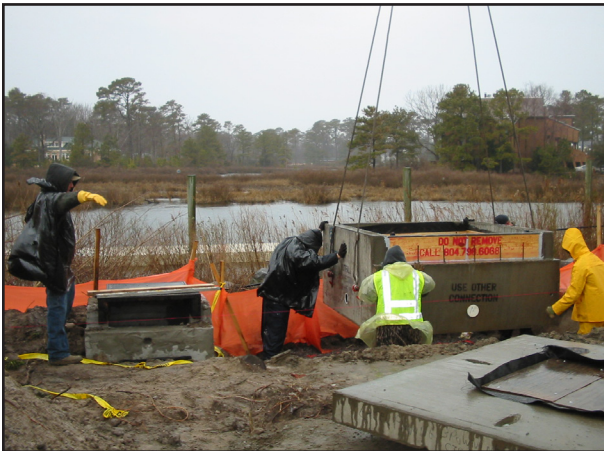
3. Filterra boxes are set in pre-prepared holes with appropriate sub-grade per plan elevations.
