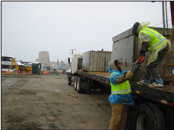
1. Filterra units shipped with top slabs separated from boxes by wooden blocks. Contractor should provide proper lifting equipment. In some cases, lifting hooks may be available.
