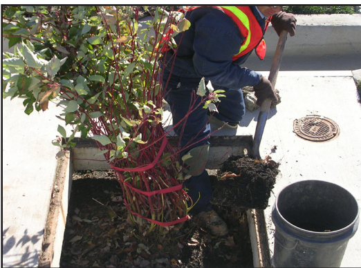
3. Removal of debris, trash and mulch
