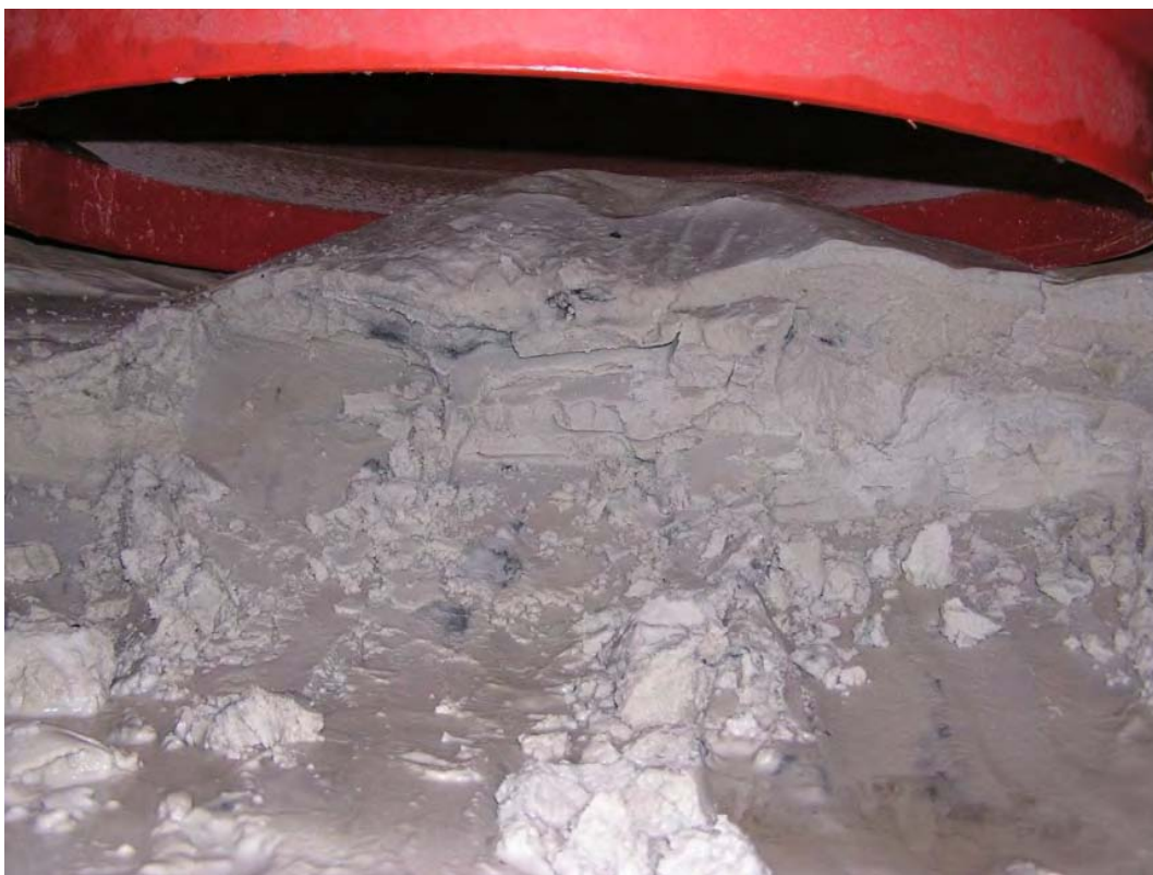
Figure 3-7: Sediment cone near Downstream Defender benching skirt
