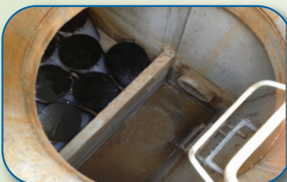
Proprietary Cartridge Filter System
