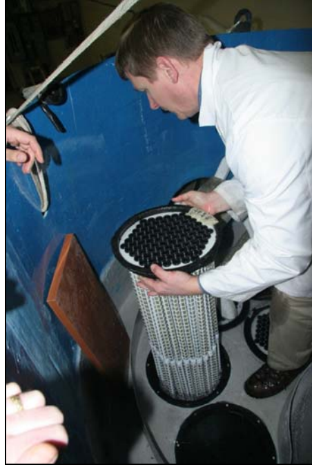
Jellyfish Cartridge Installation
