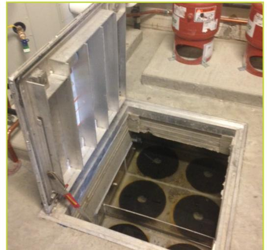
The Jellyfish Filter stops the daily laboratory concrete waste sediment from clogging the city's wastewater treatment system by removing the very fine concrete particles prior to discharge. The system design used multiple 15-inch lightweight membrane filtration cartridges. The cartridges are easily accessed at floor level by opening a hatch in small precast vaults and are designed to treat a maximum 6.94 L/s (0.25 cfs).
