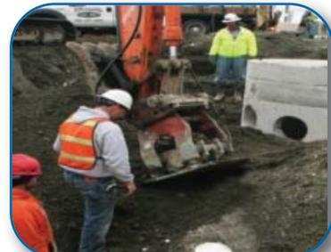
5. Set riser section(s) on the base section. Set the riser section that contains the Jellyfish Filter Deck. **Use caution and care to protect the flexible separator skirt** that will be hanging down from the Deck, as this precast section is placed.
