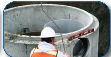
2. Set the base section of the Jellyfish Filter on solid sub-grade.
